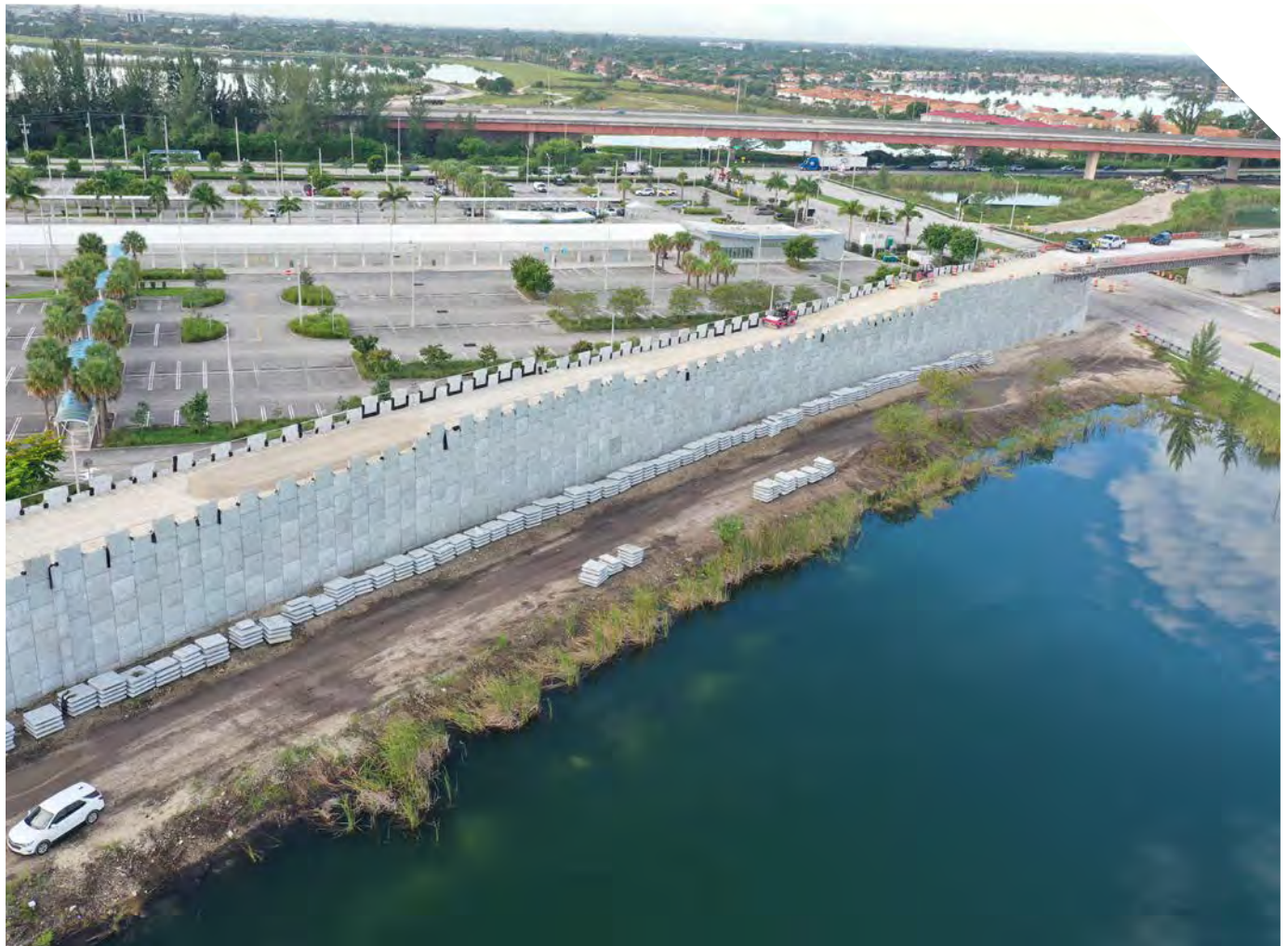
Construction of new access ramp to Telemundo Way.
