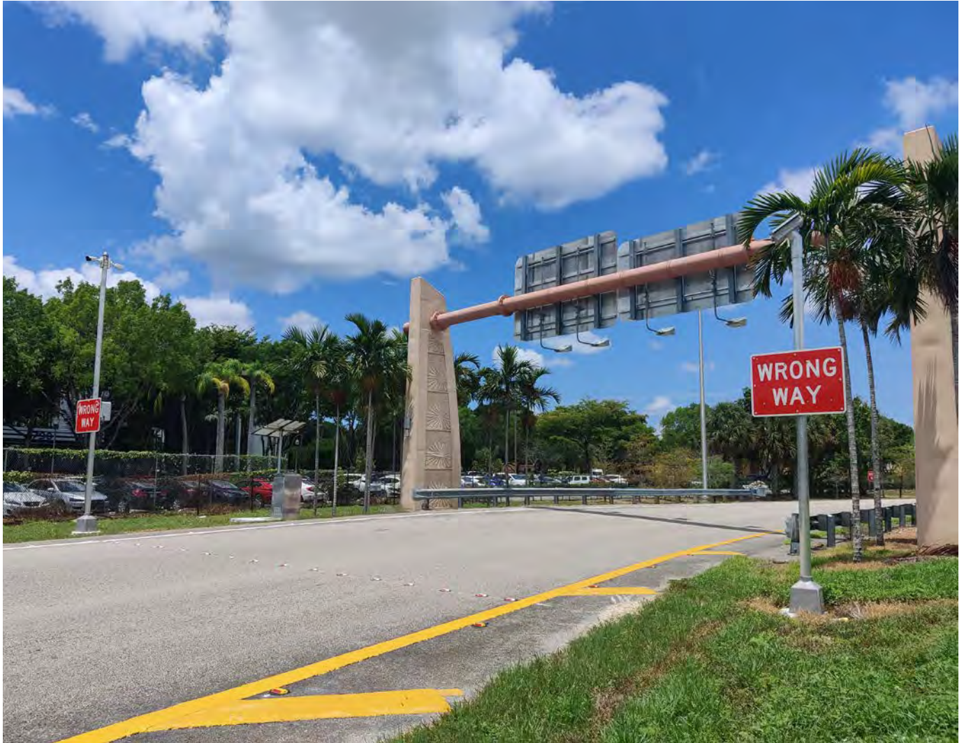
An example of the Systemwide Wrong-Way Safety Program, which includes the installation of signs; pavement markings; and systems for detecting, alerting and reporting wrong way traffic.
