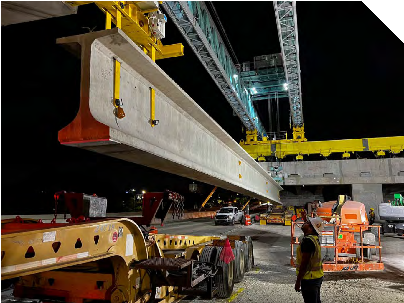
Lifting bridge beams into place.
